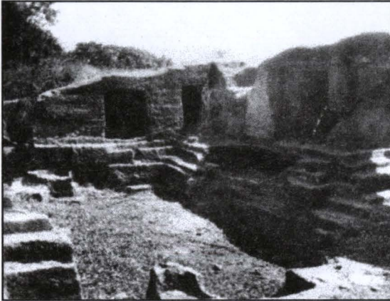
Fig 4.11; Water Tank at Magathane (Courtesy AIIS)
