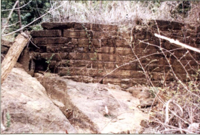
Photo 4.1: 1 st Wall of the Dam
