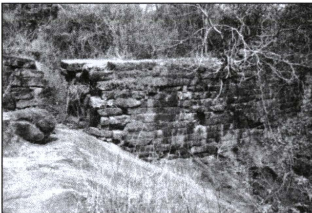
Fig. 4.2 : 2nd wall of the Dam Photo Courtesy Suraj Pandit
