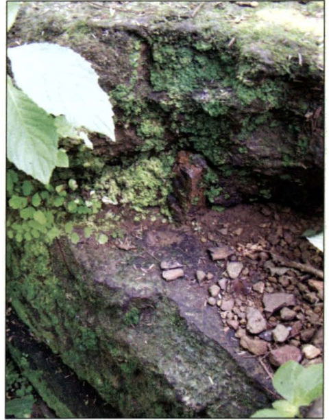
Photo 4.5: Details of the joints of the Dam
