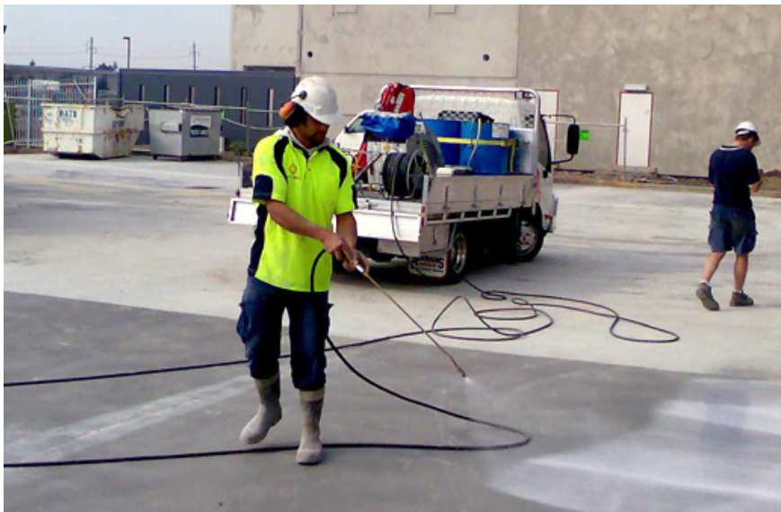
Fig 1.4: Curing by sprinkling method
