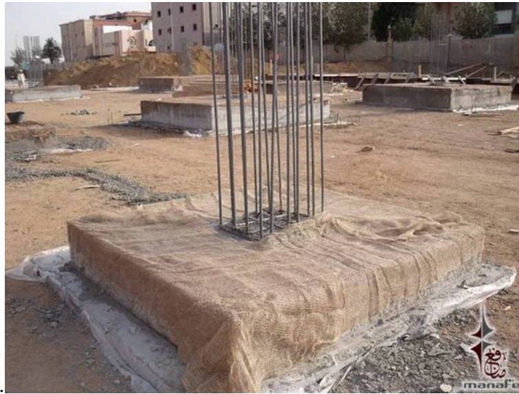
Fig 1.5: saturated wet curing
