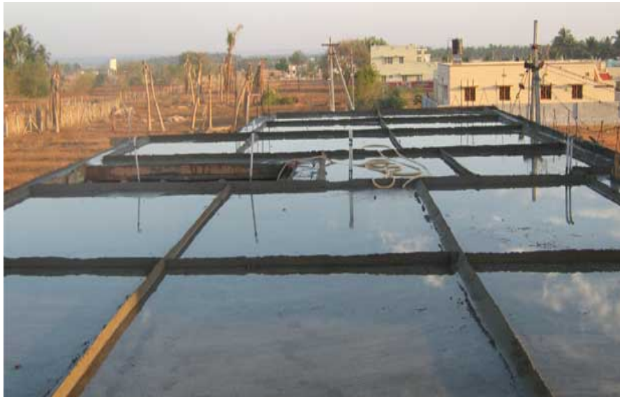
Fig1.3: Curing of concrete by Ponding
