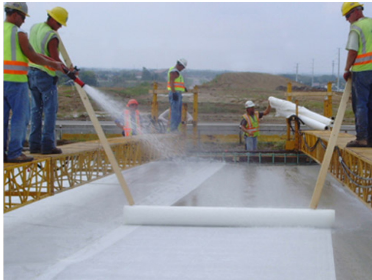
Fig 1.2: Plastic sheet curing
