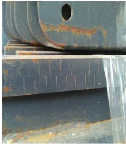
Figure1.4 Manual chiselling on trestle box
