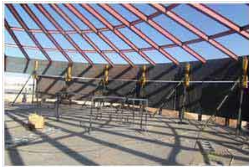
Figure1.2 Construction of storage tank
