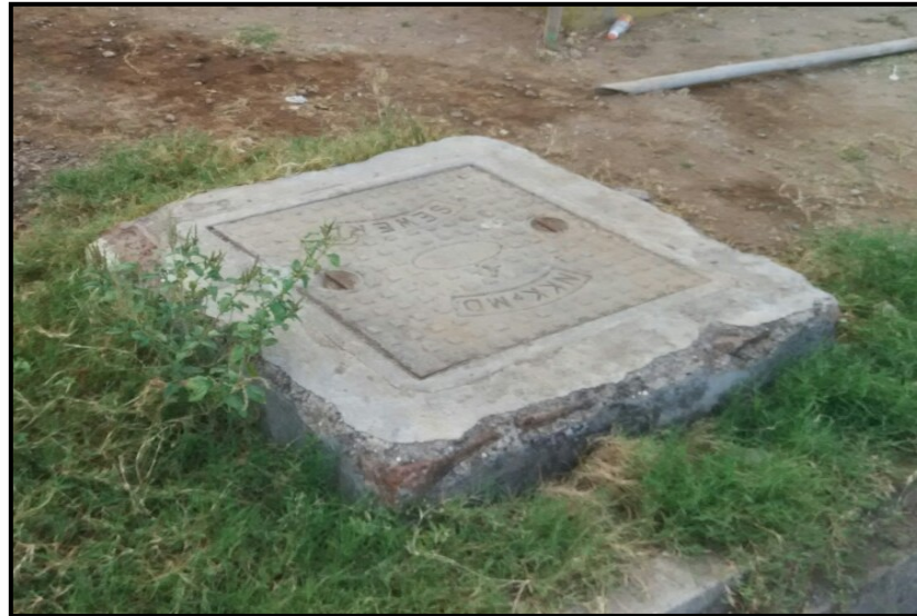
Outlet of bathroom
