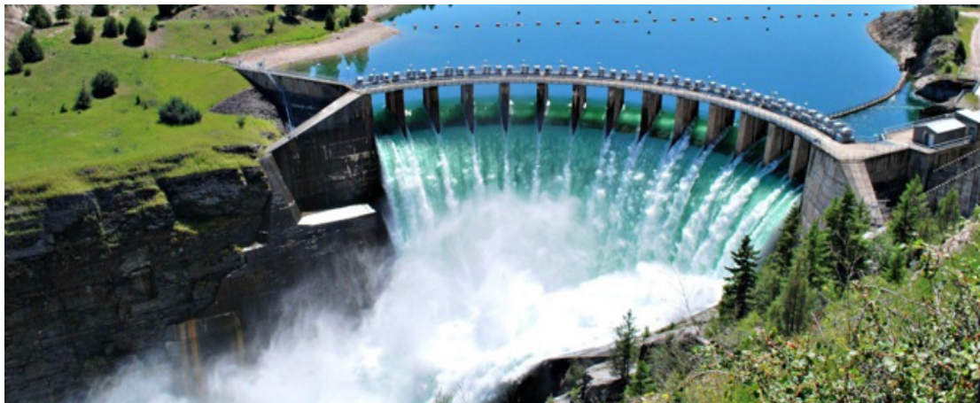
Figure 4 : huge hydro electrical dam
