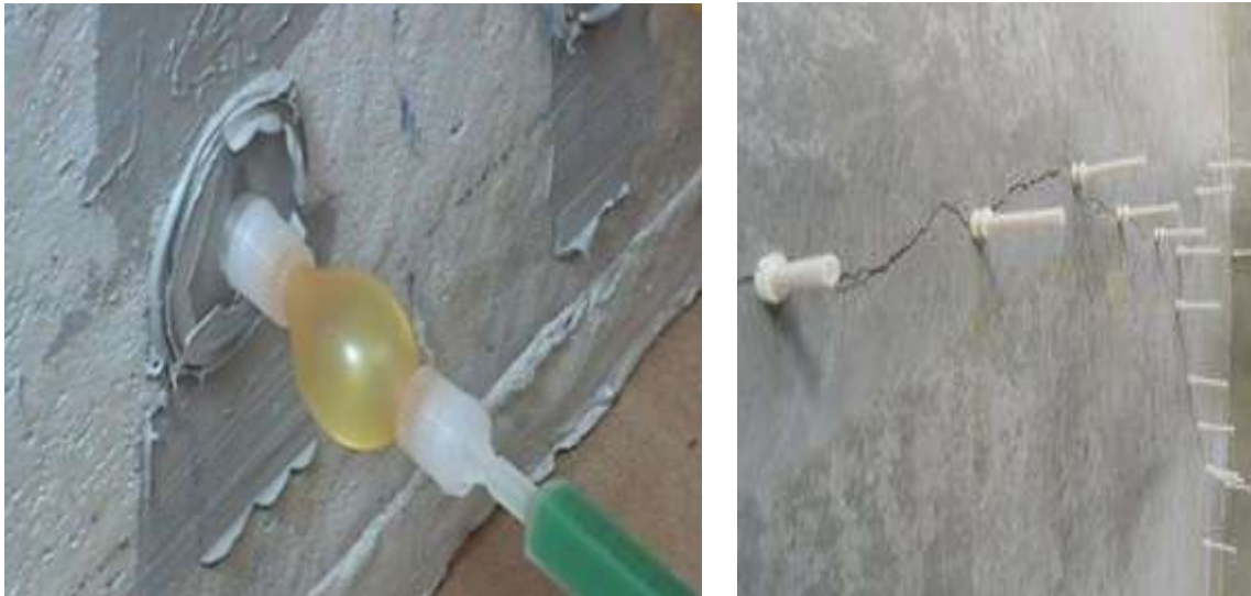
FIG 2.2 EPOXY INJECTION
