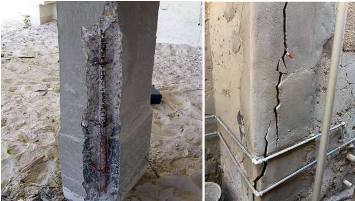
FIG 2.6 DETORiated COLUMN
