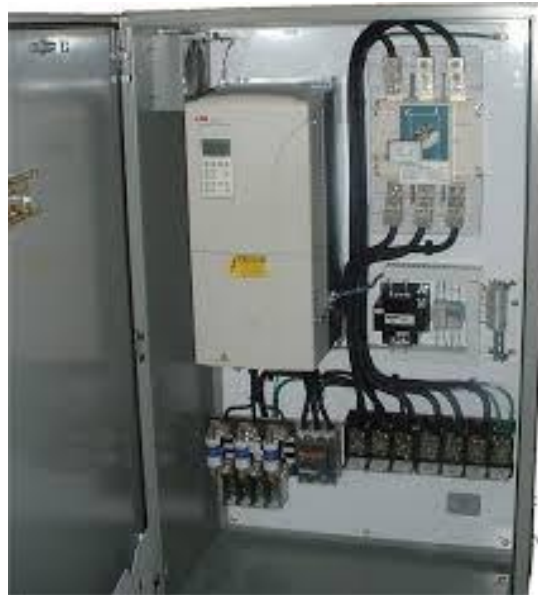
Fig. 5.3 VFD Panel
