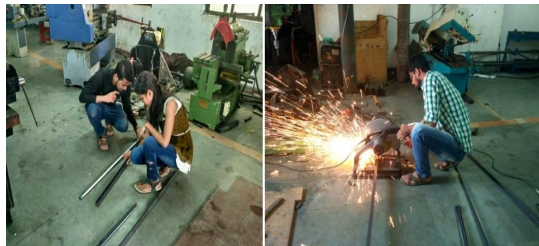
Fig.5.10 Marking and cutting of angle
