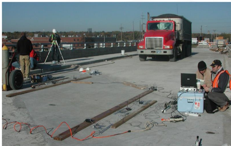
Figure 1. 5: ECC bridge deck on interstate 94, Michigan (Source: MDOT research, 2008)
