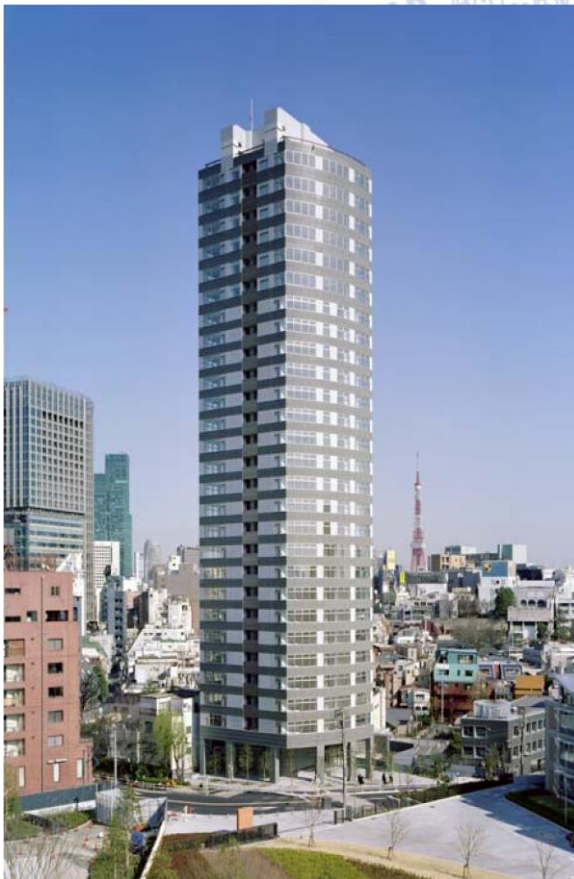
Figure 1. 4: Glorio Roppongi high-rise residential building, Tokyo (Source: www.cif.org )
