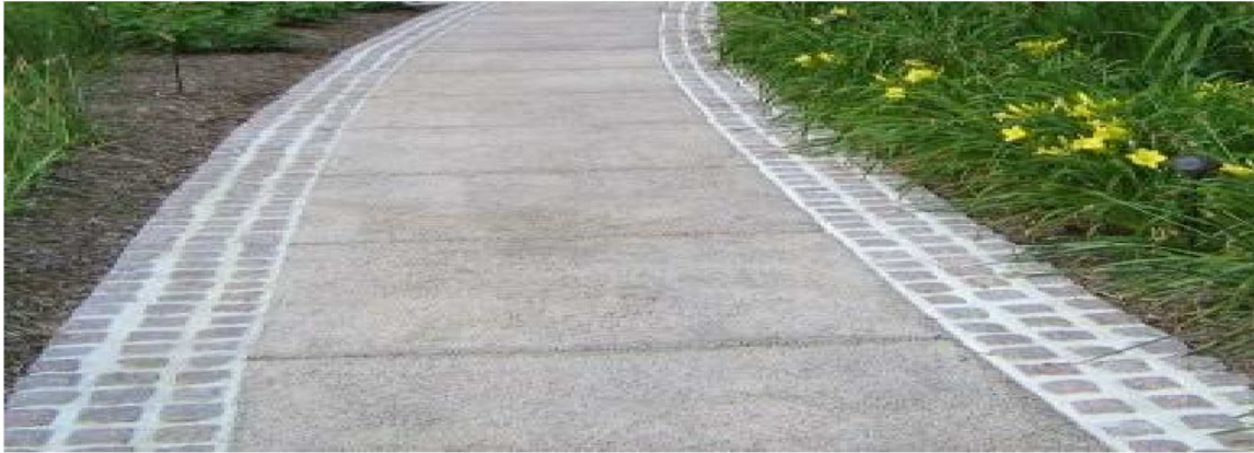
Fig 2: Pervious concrete walkways
