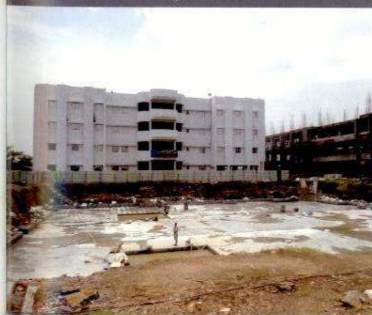
Work in Progress of AIKTC
