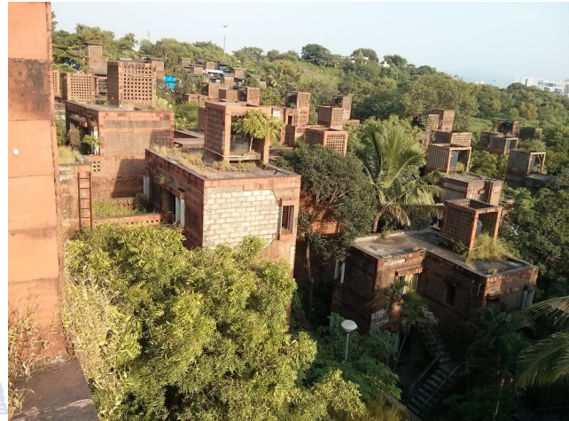
Figure5. 1 View of housing CIDCO
