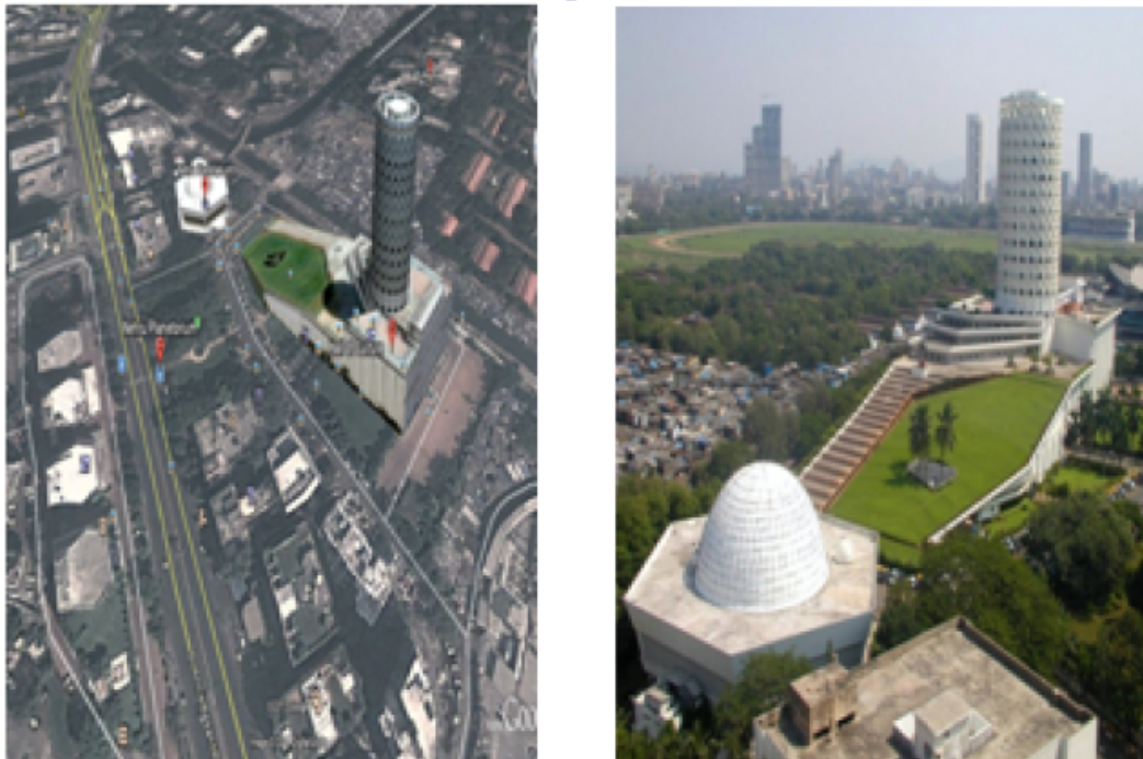
Figure9. 1 Google image bird's eye view of the structure
