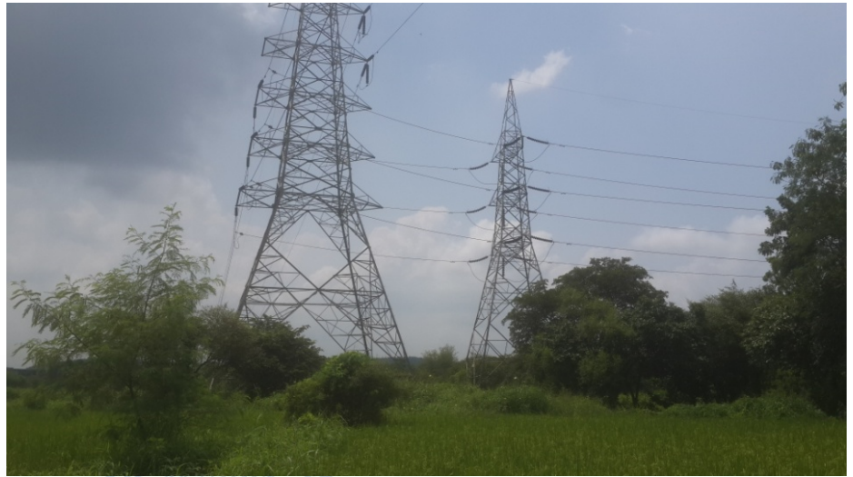
Figure11. 10 There are 2 high voltage wire touching the site
