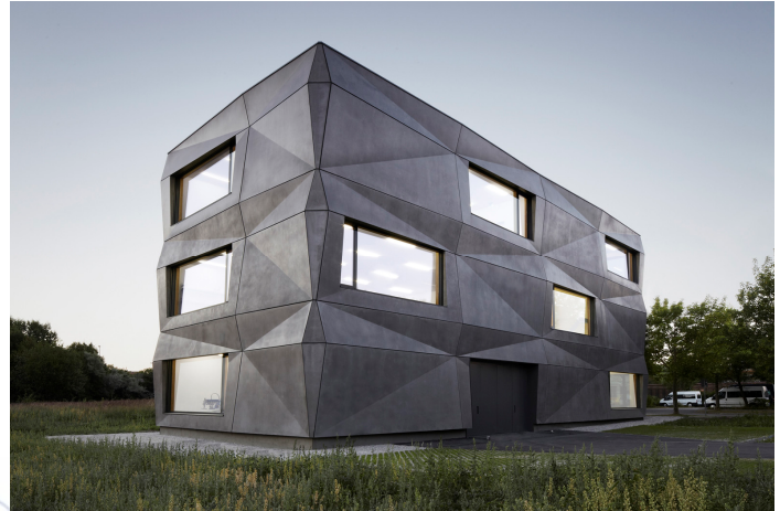
Figure4. 1 View of the structure
