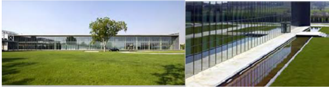
FIGURE8. 13 External view of the building and north west facade
