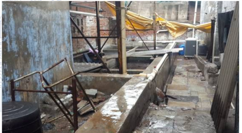
Figure1. 6 Washing area after dyeing.
