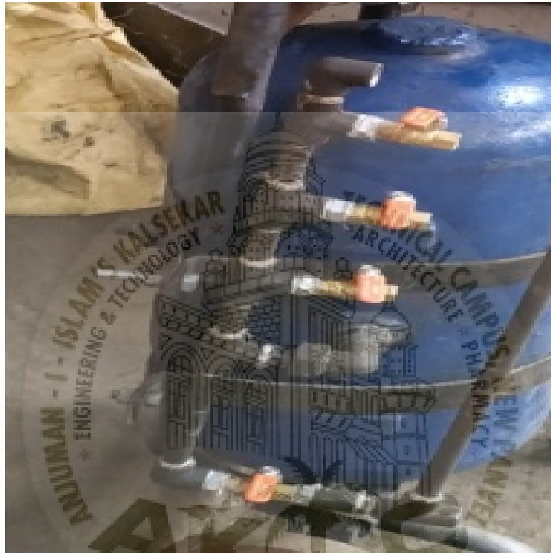
Figure 4.8: Piping Arrangement For Isolating Cocks
