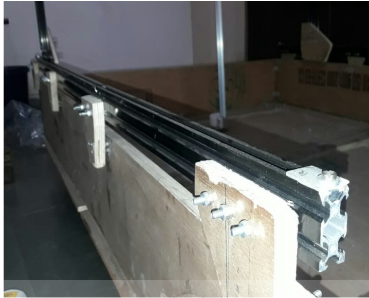
Figure 4.35: Placing of Aluminum Extrusions
