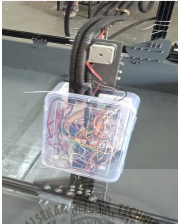
Figure 4.47: Placing of Farm-Dino and Power Supply Box
