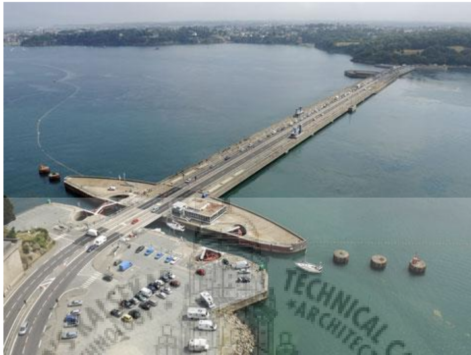
Figure 2.2 The first tidal power plant in Rance (France) also used as bridge
