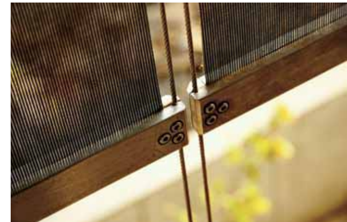
Astral Corporate House has a unique louver system made of fabric, developed by the industrial design team at HCP as an almost diaphanous filter for light, creating a glare-free environment by diffusing strong daylight
