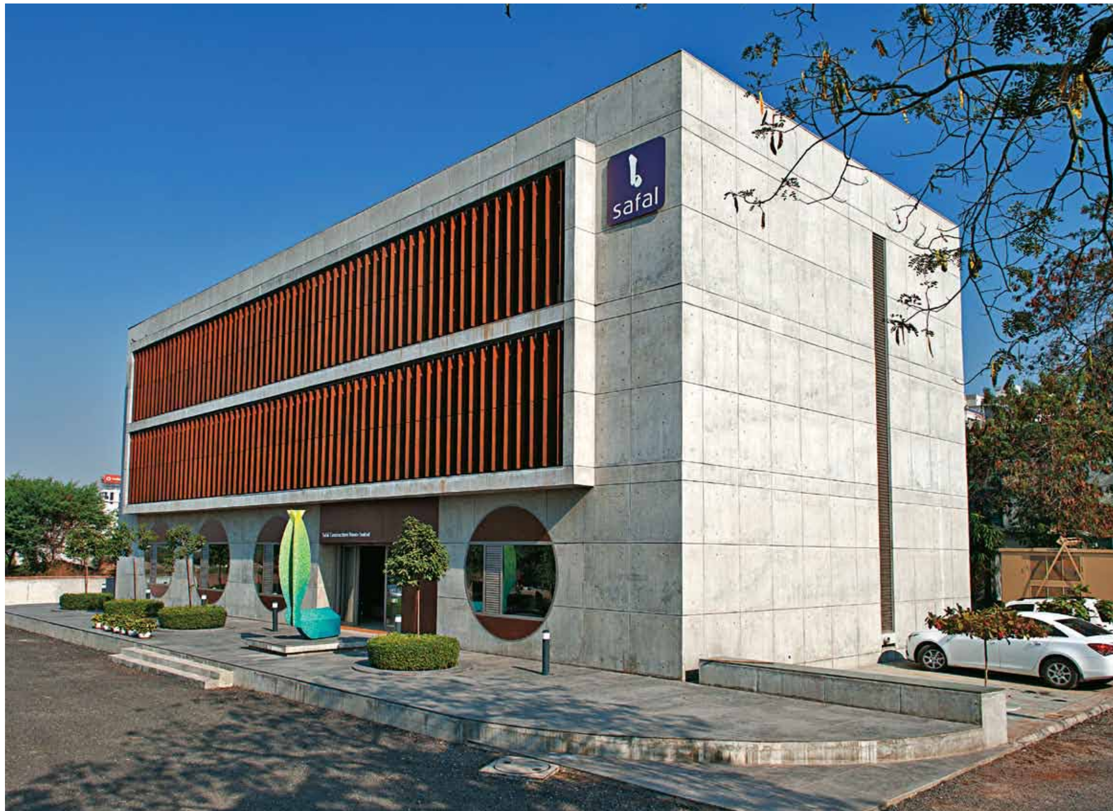
HCP have employed technology as a powerful aesthetic device to define the architectural language of Safal Corporate House
