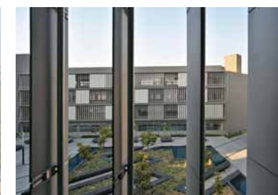
↑ Manually adjustable louvers allow for a great degree of flexibility in controlling the interior environment, both in terms of light and air circulation
