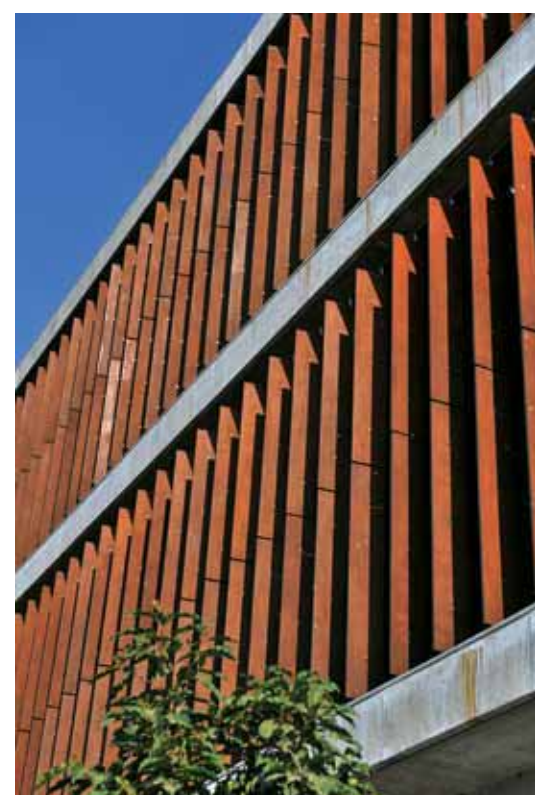
The space between the vertical rigid louver system and the inner skin controls the heat accepted by the building; the flexibility built into the plywood system allows for configurations to suit the visual and climatic dimensions of the building
