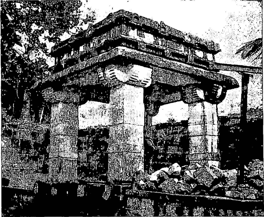
Plate I " Vīṣamaṇḍapika, Mallikārjuna Temple, Mahākūṭa, Ca. early 7th Century. View from the ground level".
