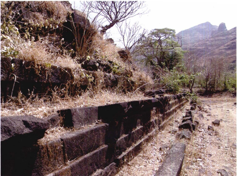
Fig. N 2 . 2 - Closer view of Plinth
