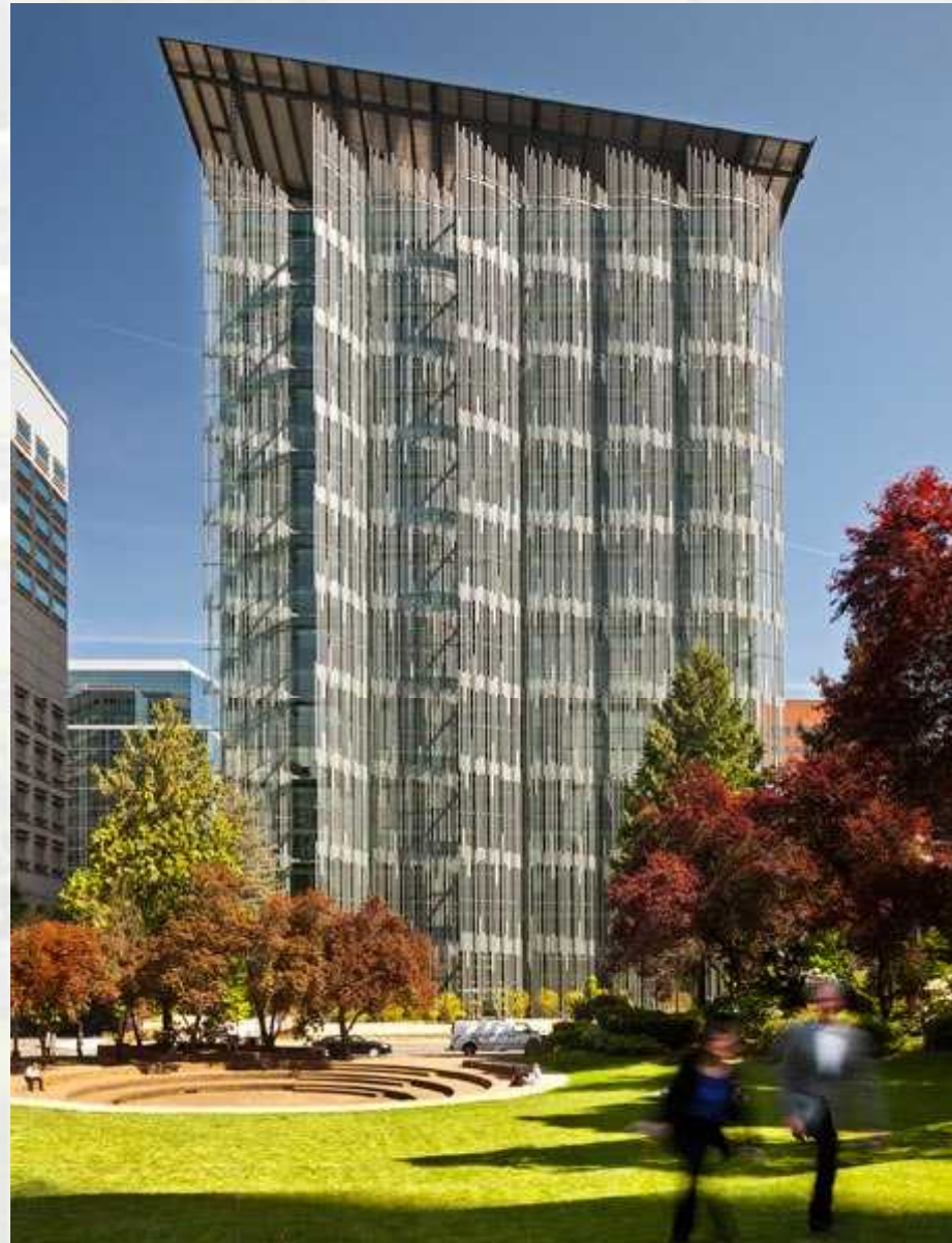
EDITH GREEN-WENDELL WYATT FEDERAL BUILDING MODERNIZATION, PORTLAND, OREGON
