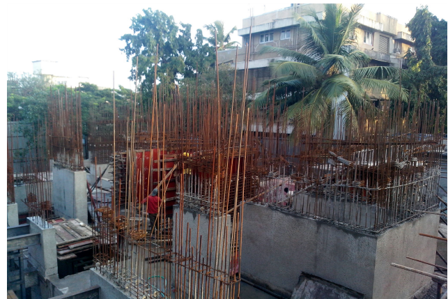
Fig -2: Concrete filling at level 1
