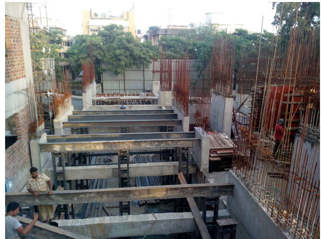
Fig -1: laying of slab bottom at site
