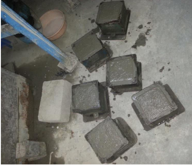
Fig: 3.5: Placing of Concrete.
