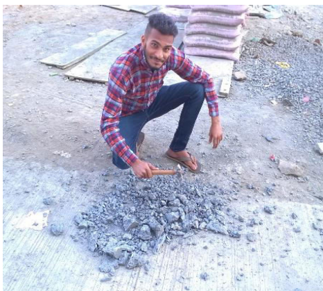
Fig 3.2: Crushing of debris
