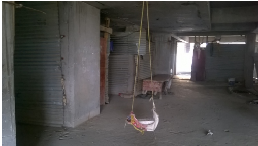
SHEDS INSIDE THE UNDER-CONSTRUCTION BUILDING.
