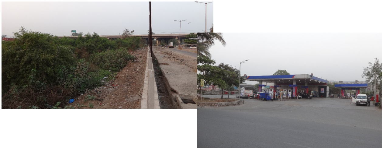
PATROL PUMP ON THE SITE
