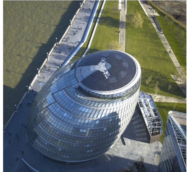
USE OF SOLAR PANEL ON THE ROOF
