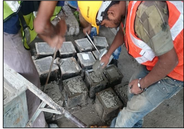
Figure 4.2 Tamping of concrete
