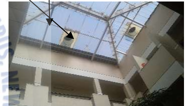
courtyard with skylight
