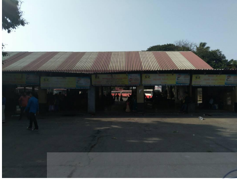
Fig. No.40. showing Waiting area (Mumbai route bay)
