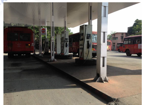
Fig. No.57. showing Fuel pump machine and buffer space where a person can stand
