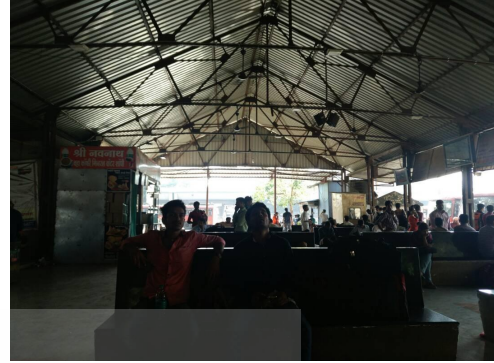
Fig. No.41. showing Inside of Waiting area (Dark Area)
