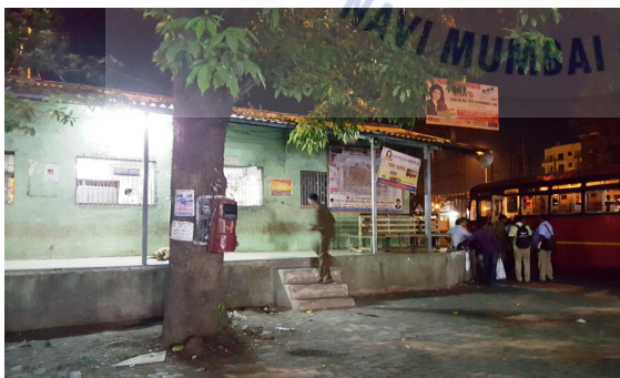
Fig. No.44. showing Ticketing Block (Night View)
