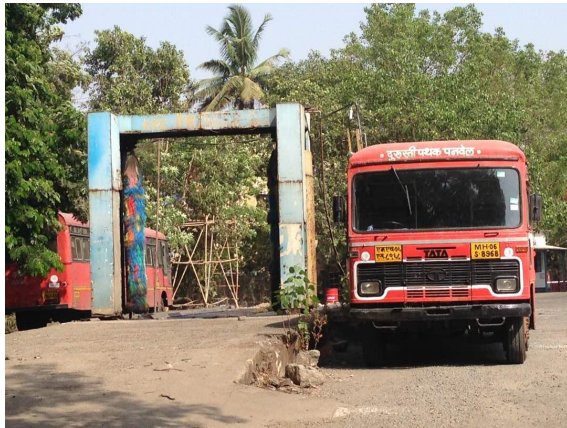
Fig. No.52. showing bus washing tower
