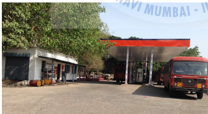
Fig. No.56. showing Fuel Pump with Cabin
