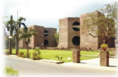
Figure 73 : Building façade of IIM
