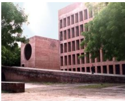
Figure 91 : Building façade of IIM
