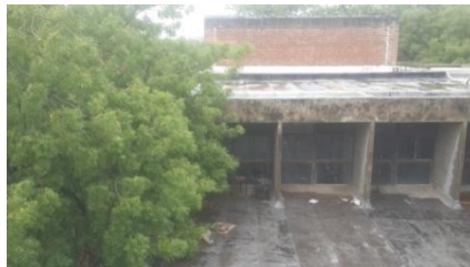
Figure 70 : Façade of the building covered with trees
