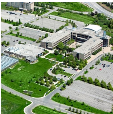
Figure 141 : Aerial View of Glendale Campus
