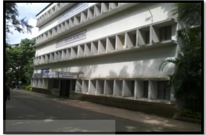
Figure 23 : Fin and box section in Elevation
