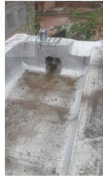
Figure 72 : water channels at the roof
