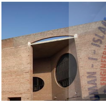
Figure 83 : Façade of the building
