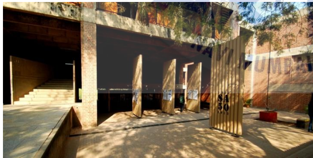
Figure 56 : Facade of the building
