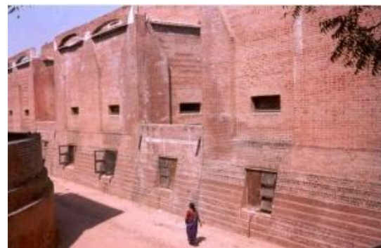
Figure 92 : Lower windows for ventilation
