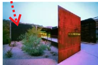
View of the structure
