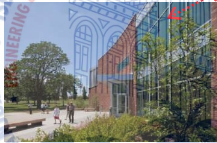
The hardscape merges with the structure and acts as a Spill out
