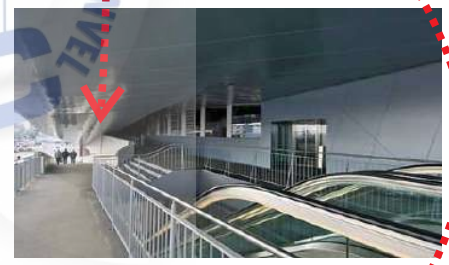
View of the bridge and structure
