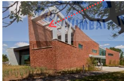
Material contrast of Zinc and Brick
