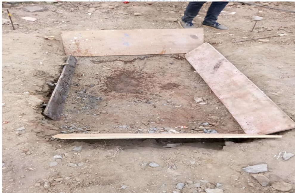
Fig 3.2.4.2 Compost Pit after excavation
