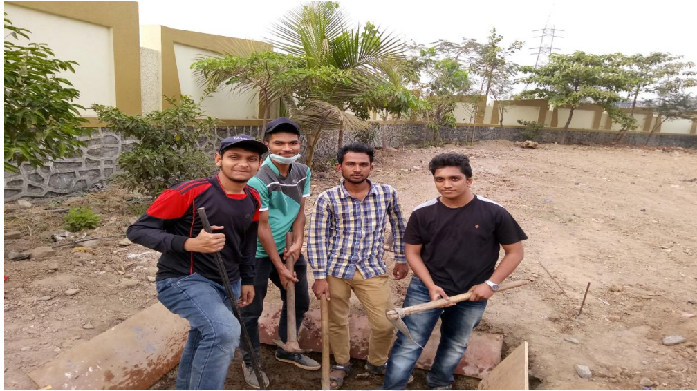
Fig 3.2.4.3 During excavation of Pit
