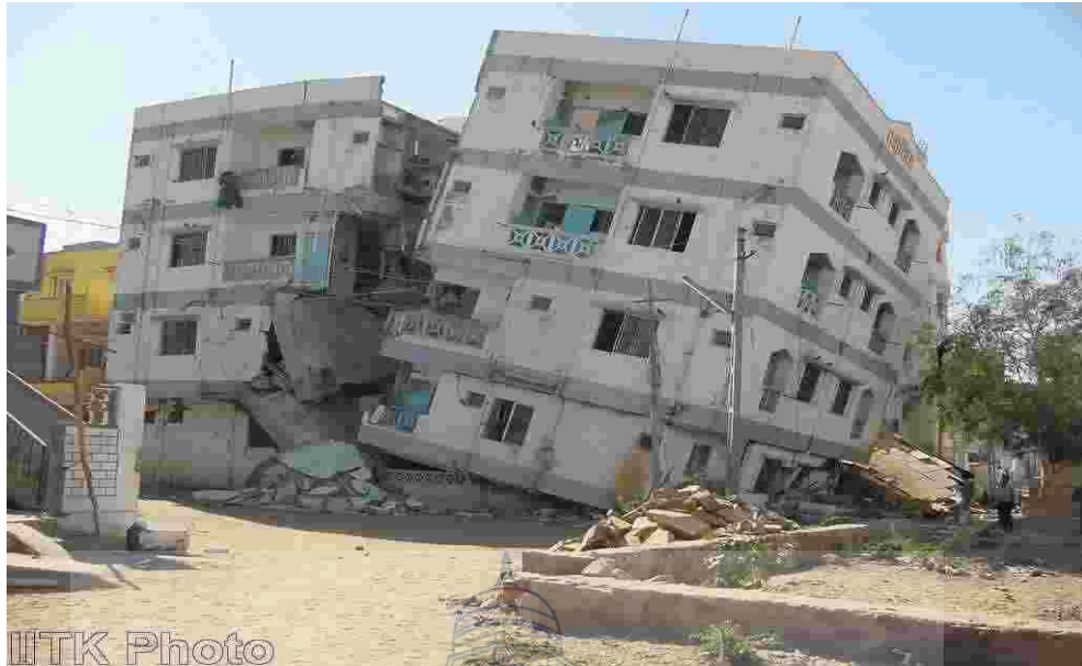
Figure 2.4 Failure of Approximately Similar Buildings During Bhuj Earthquake 2001 [IITK]
