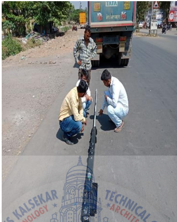
Fig 4.15: Recording of Benkelman Beam deflection reading
