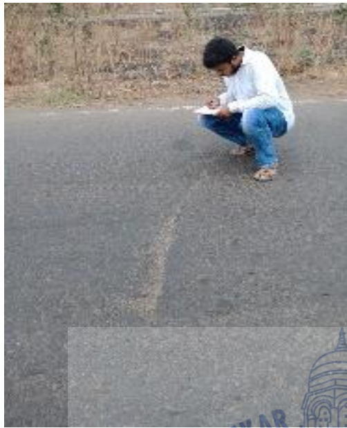
Fig 4.3: Patching on selected pavement surface
