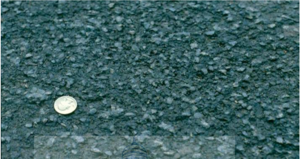
Fig 3.7: High Severity Ravelling Of Asphalt Surface
