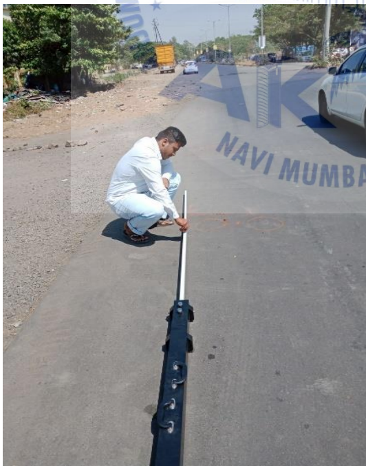
Fig 4.13: Setting of Benkelman Beam
