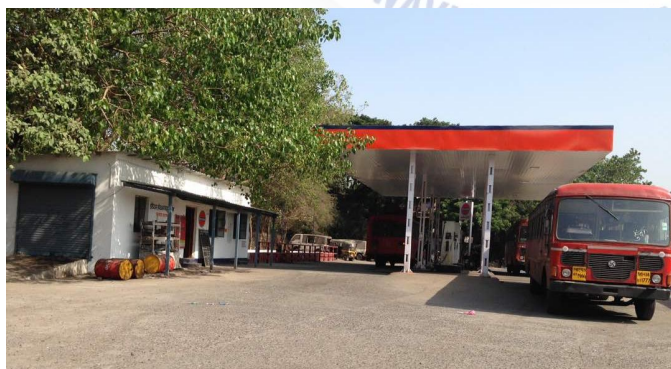
Fig. No.56. showing Fuel Pump with Cabin
