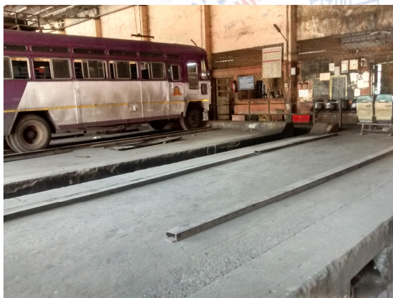
Fig. No.48. showing Pit Area in Garage
