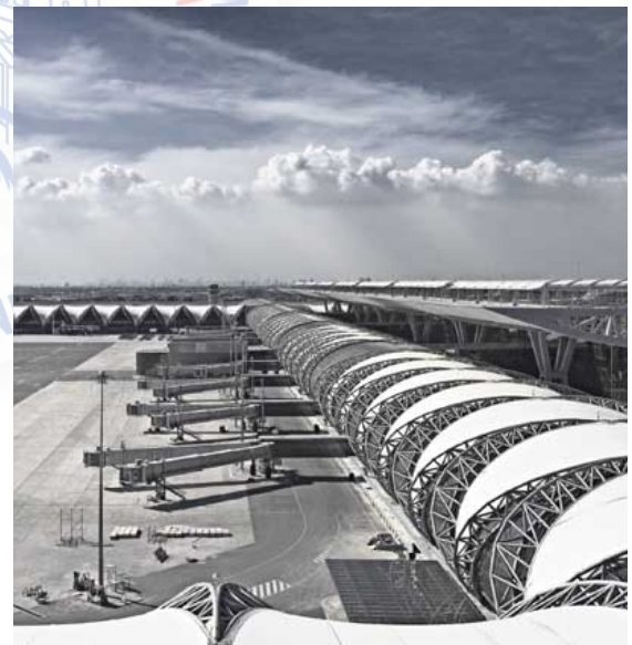
Fig (2.36) Suvarnabhoomi Airport
