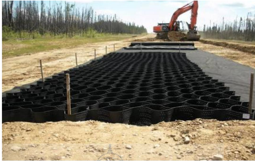
Figure 3.4.6 Stabilization by Geo-Textiles
