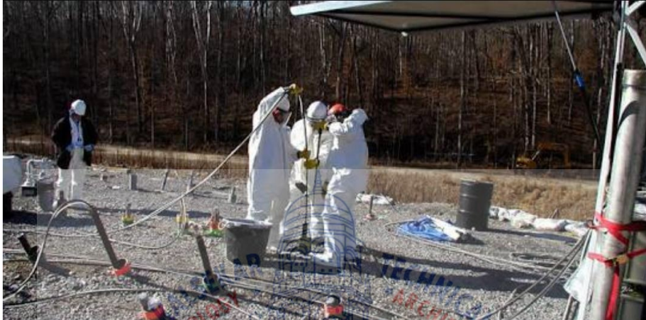
Figure 3.4.5 Stabilization by grouting
