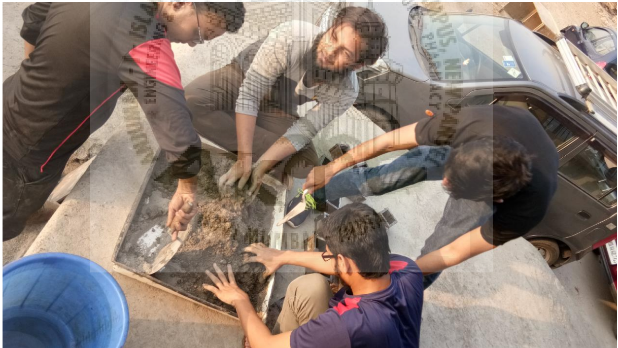
Fig 4.2: Direct mixing of bacterial solution in cement mix
