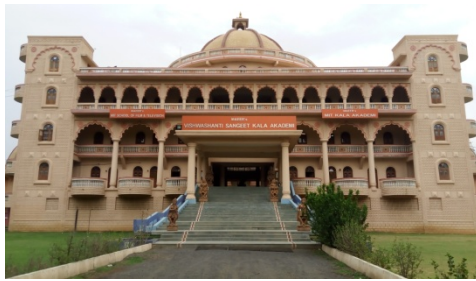
Figure 5 Entrance, Admin Block and Hostel Block
