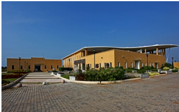
Figure 30 Main Building Entrance
