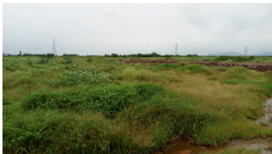
Figure 83 Approach road under construction
