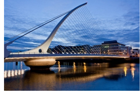
Figure 88 The Harp Bridge by Santiago Calatrava
