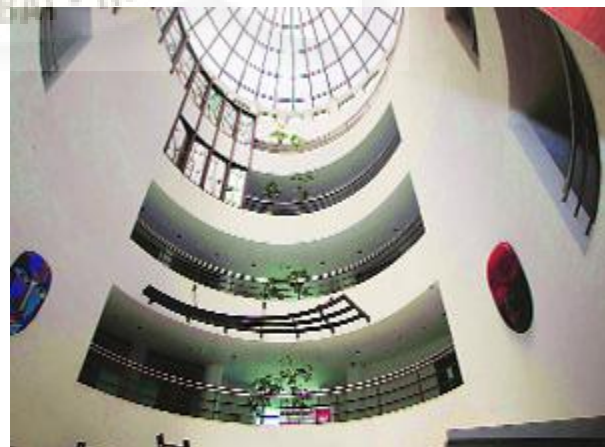
Figure 27. Image showing skylight in block A
