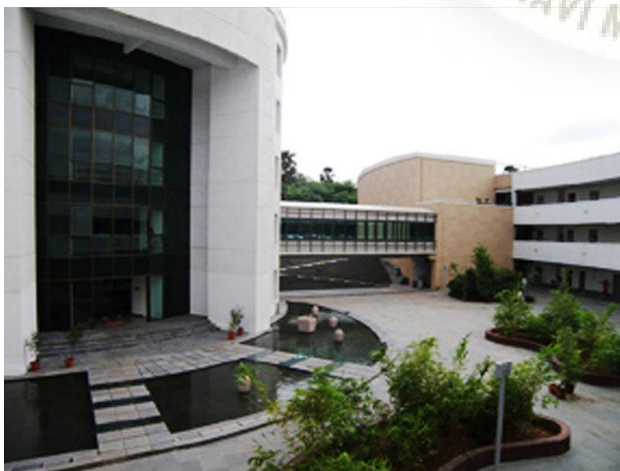
Figure 26. Image showing connecting bridge
