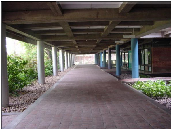
Figure 50. Images showing source of ventilation in structure (NID)
