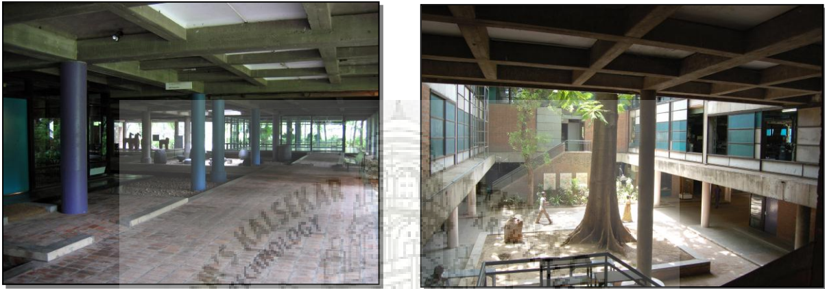
Figure 51. Images showing light fixtures
