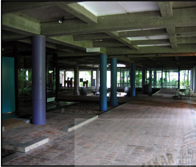
Figure 40. Image showing Structural detail
