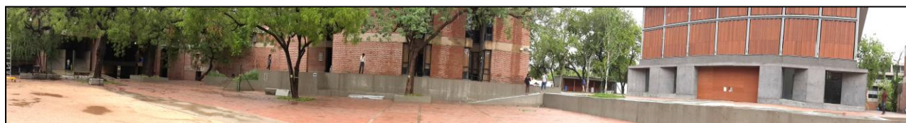
Figure 62. Panoramic view of central courtyard
