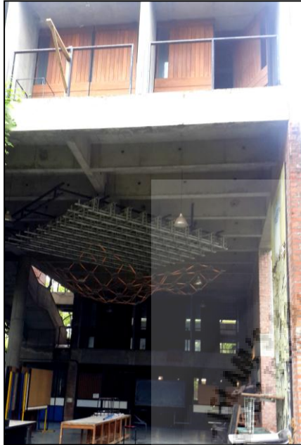
Figure 61. Image showing material of structure (RCC)
