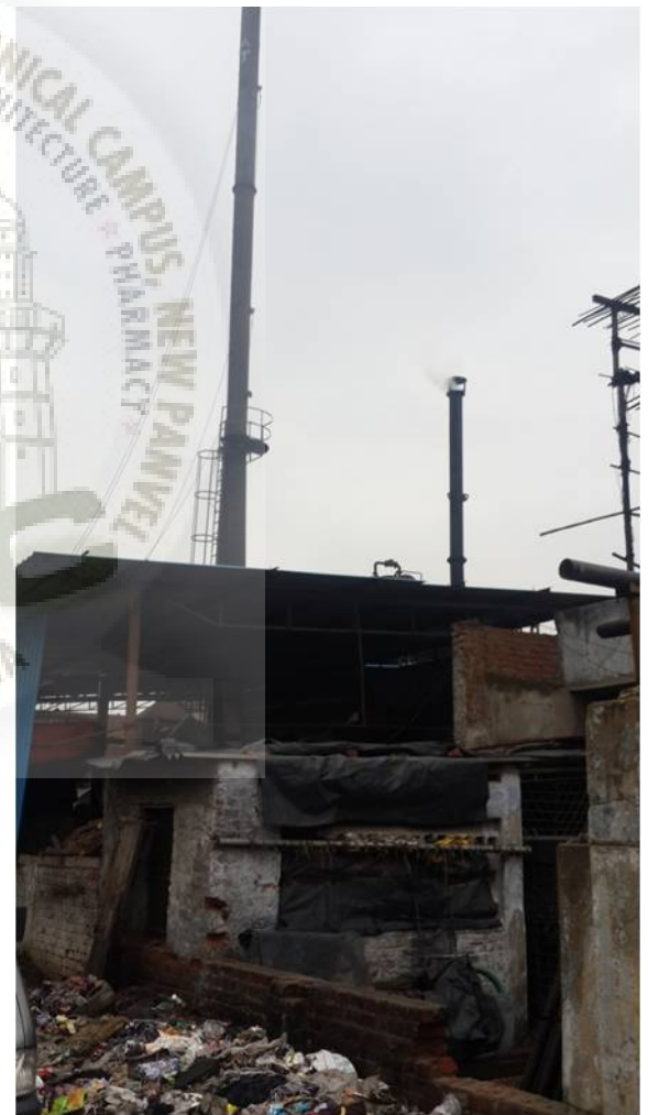
Figure1. 21 View from the entrance
