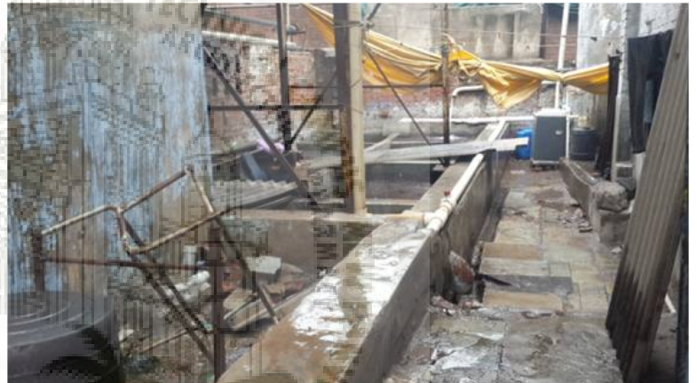
Figure1. 6 Washing area after dyeing.
