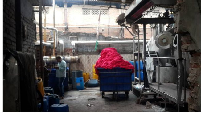
Figure1. 9 Boiler and dyeing area.
