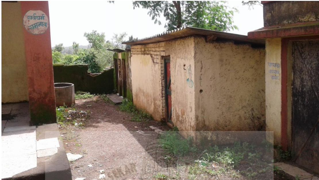
The toilet block for girls
