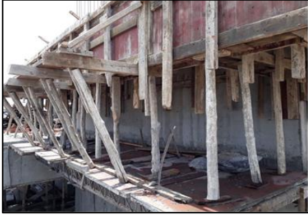
Figure 4.4 Shuttering Work (A-Building)
