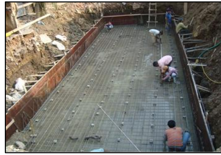
Figure 4.5 Raft Footing (B-Building)
