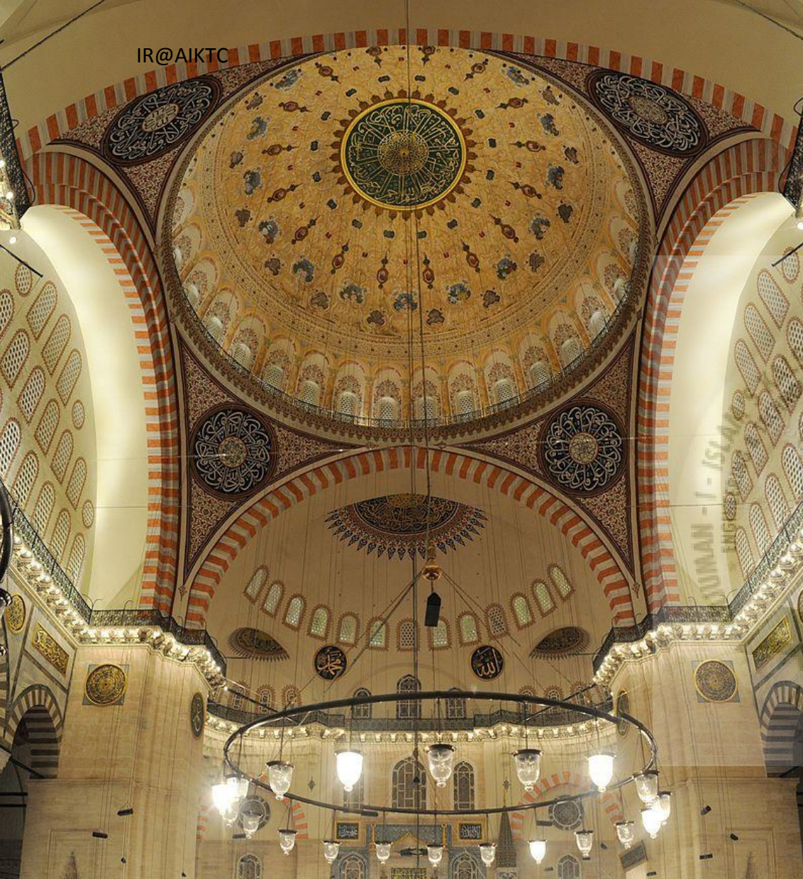
The Suleymaniye Mosque Istanbul (1558): The series of openings in the dome present for sound absorption Service By KRRC (Central Library)
