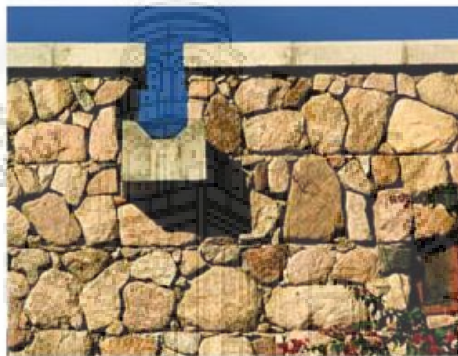
RAINWATER SPOUT DETAIL
