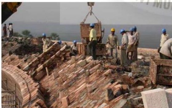
Filling the back with random masonry
