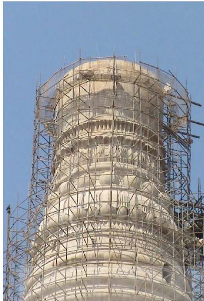
Conical dome in progress
