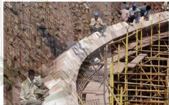
Interlocking stones of the main dome
