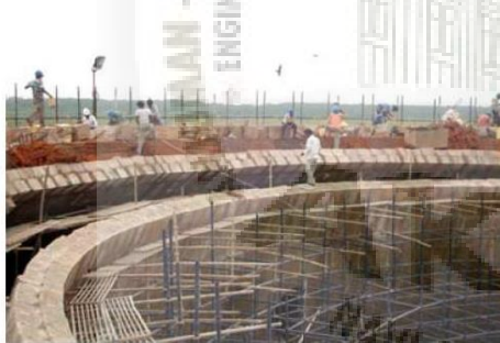
Auxilliary dome near completion
