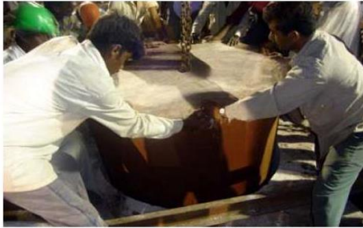
Laying the keystone of the main dome
