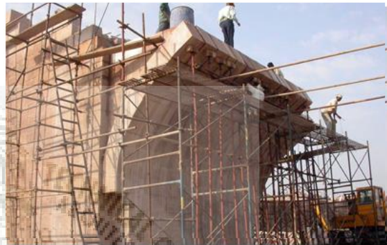
Building the entrance vault, corbelling without formwork
