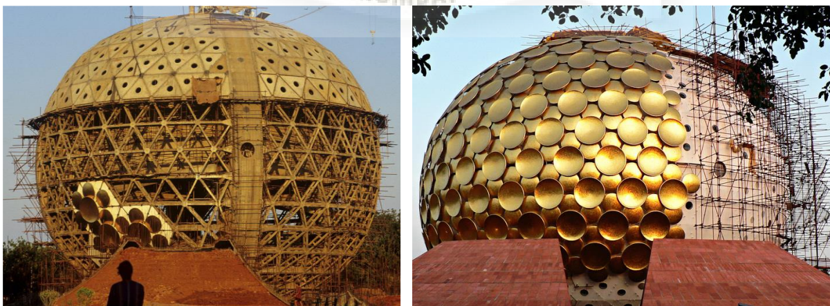
Figure 41 Phase 3 and 4 of construction
