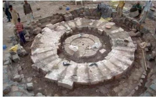
Main dome completed
