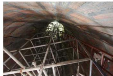
Conical dome being completed
