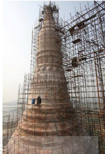
Conical dome towards completion
