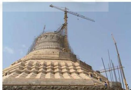
Catenary dome in progress
