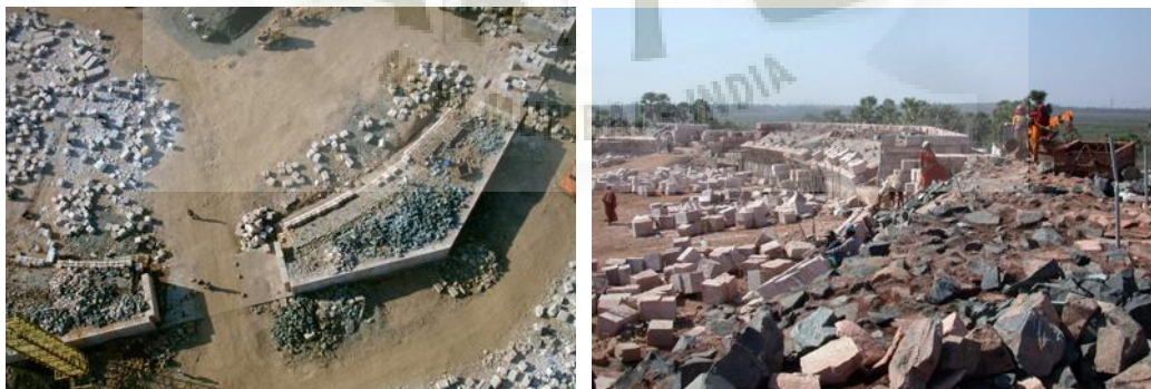
Figure 64 Begging of construction
