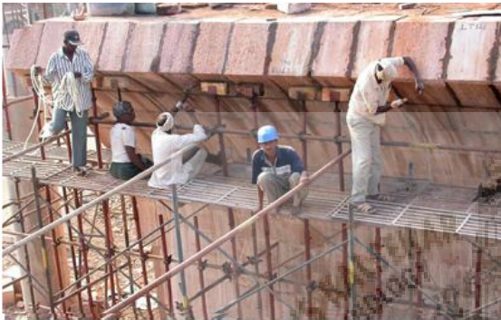
Building the entrance vault, corbelling without formwork
