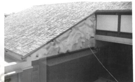
Pop and compressed earth blocks wall after finishing.
