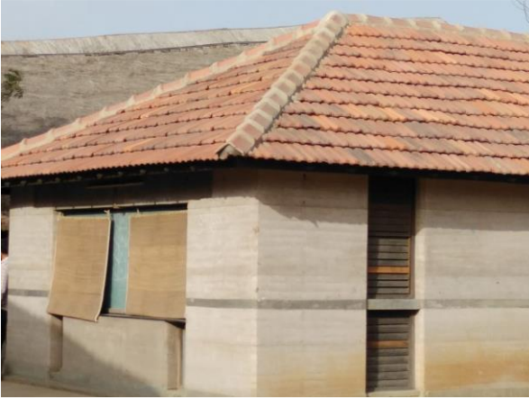
Image showing the Mangalore tiles used as a roof cladding.
