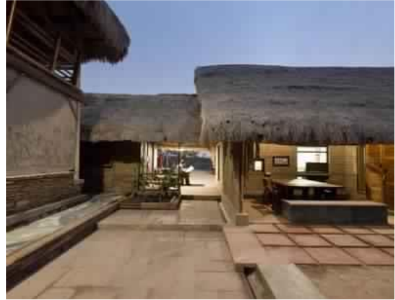
Image showing the entrance to the structure.
