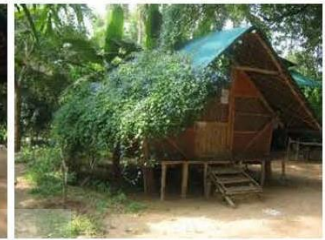
Guest house, front view
