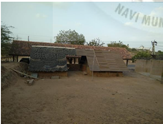
Image showing the experimentation done on the roofing using type rubber.
