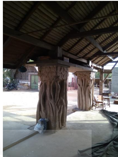
Image showing the precast column.
