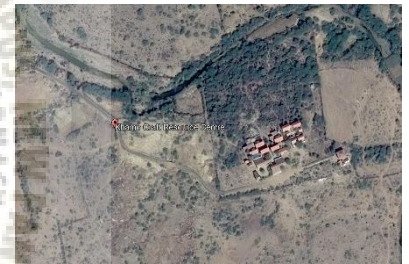
2015-The project got completed.
