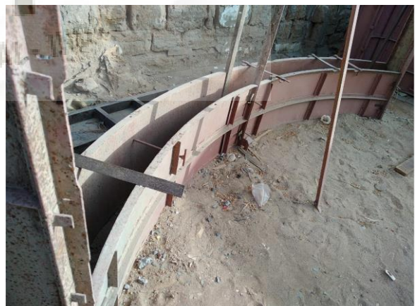
Image showing the rammed earth mould
