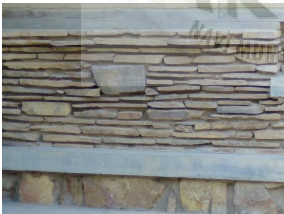
Image showing the stone rubble masonry
