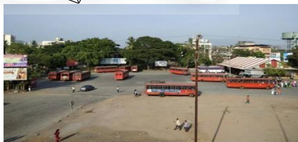
Bus Circulation Area
