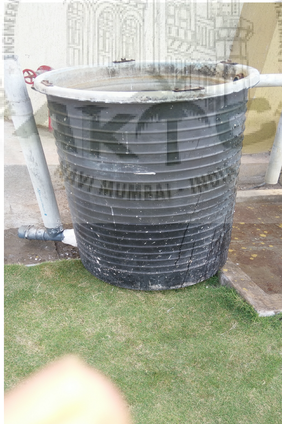
Figure 5.1: Digester Tank
