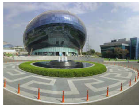
LEED Platinum is the highest level of green rating for buildings and with this recognition, the Infosys Pune campus becomes the largest in the world to achieve this distinction.
