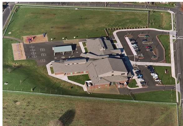
C5.FIG.3 ACTUAL ARIEL VIEW OF THE SITE AND ADJOINING COMMUNITY FIELD
