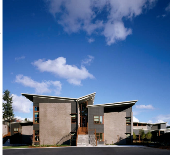
C5.FIG.1 VIEW OF ONE OF THE SCHOOL CLUSTERS
