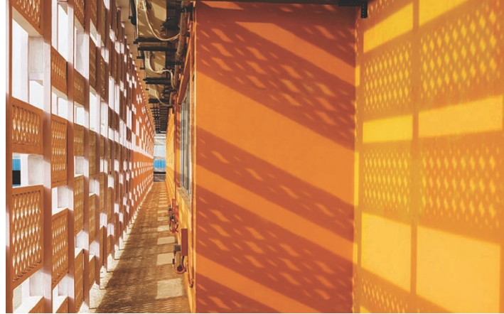
C1.FIG.7 VIEW OF THE BUILDING SKIN AND THE WALL CREATING A BUFFER SPACE FOR THERMAL COMFORT
