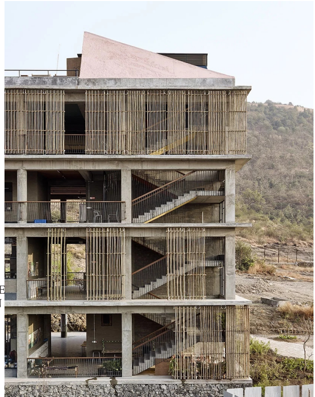
C3.FIG.2 THE CONCRETE STRUCTURE HAS BEEN LEFT OPEN WITH ONLY BAMBOO SHADING TO PROVIDE A SENSE OF ENCLOSURE
