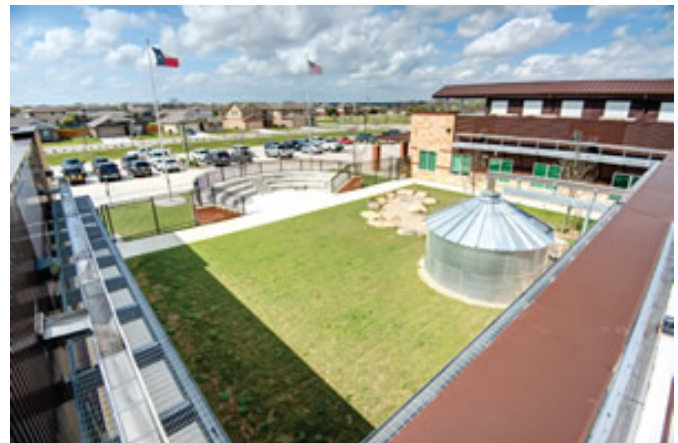
Fig.22. grey water system at howard norman elementary school
