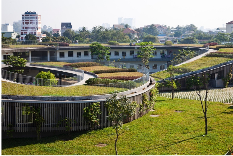
Fig.24. green roof and landscape merging at farming kindergarten, Vietnam
