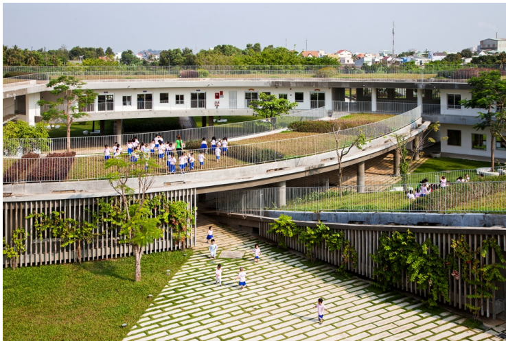
C4.FIG.2 THE BUILDING'S CONTINUOUS GREEN ROOF CONTAINS BENEATH IT ALL OF THE SITE'S DIFFERENT PROGRAMS
