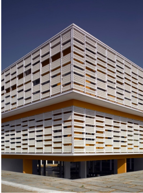
C1.FIG.6 VIEW OF THE BUILDING
