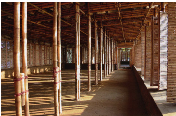
Fig.27. use of contextual and vernacular materials at METI SCHOOL, BANGALADESH
