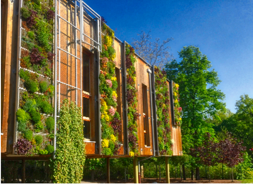
Fig.29. Example of vertical green skins farming and aesthetics at school façade in France
