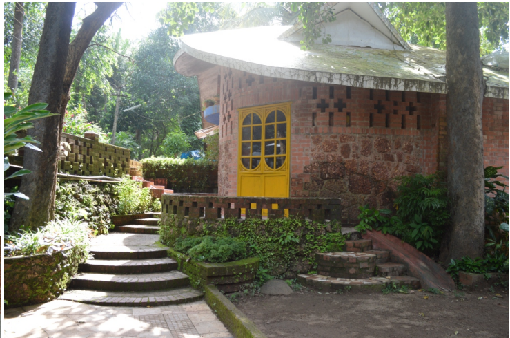
C7.FIG.1 VIEW OF THE SCHOOL
