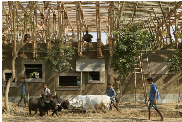
C6.FIG.5 USE OF LOCAL LABOR AND MATERIALS
