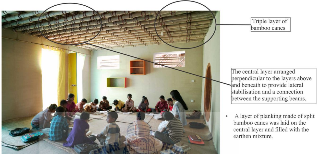
Figure-5.11 Showing Roof Details
