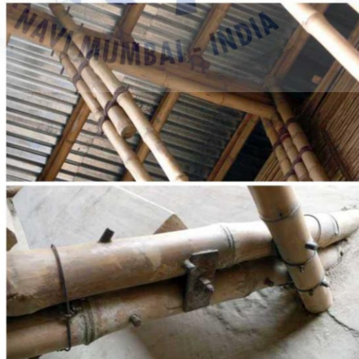
Figure-5.9 Showing Joinery Details
