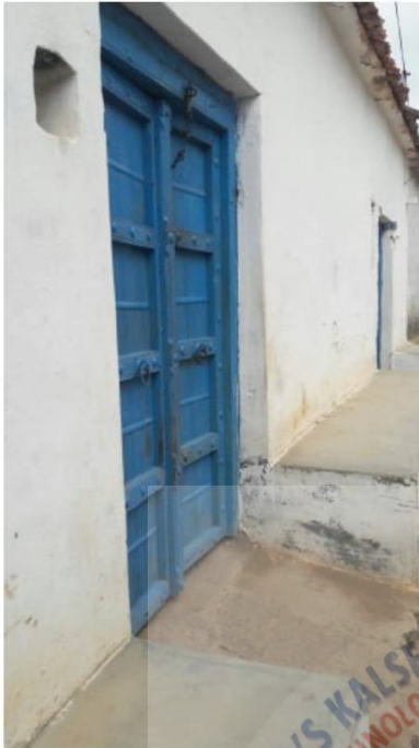
THE HOUSES ARE PLASTERED WITH LIME
