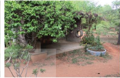
C2 Figure No:19 ACCESS TO BACKYARD FROM MATHS ROOM
