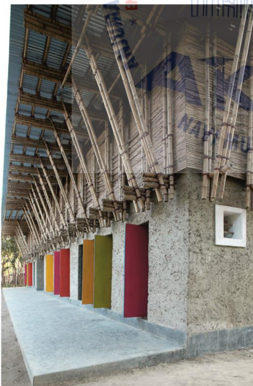
C6.FIG.3 USE OF VIBRANT COLOURS AND SUSTAINABLE MATERIALS IN THE END WALL DETAIL
