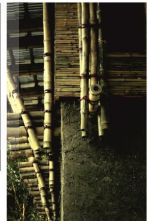
C6.FIG.23 THICK WALLS ASSURE A COMFORTABLE CLIMATE ON THE GROUND FLOOR OF THE BUILDING.
