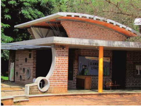
C2 Figure No:02 FILLER SLAB TECHNIQUE USED IN PLAY ROOM .
