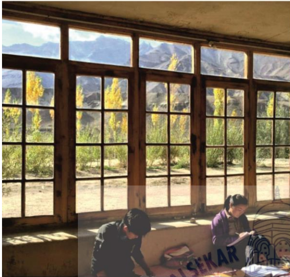
C5 Figure No:16 NATURAL SUN LIGHT IN CLASSROOMS
